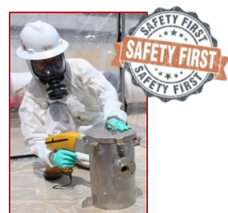
Mercury decontamination of process equipment
